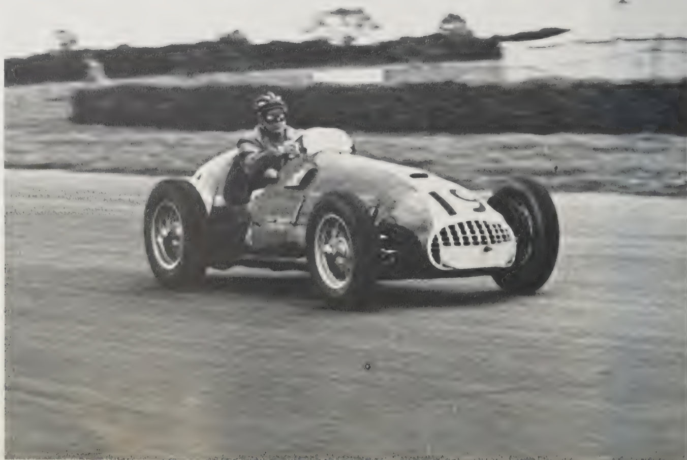
Preceding pages: Type 500F2 at Bremgarten (Swiss Grand Prix, 1953). The large bulge was necessary for the longer carburettor intakes
